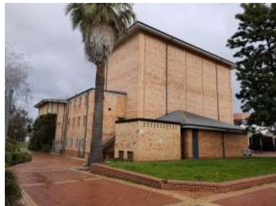
Figure 2-4: Looking south-west at the site from Swift Street, showing the theatre and vehicular access
