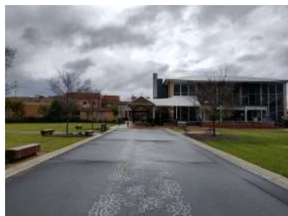
Figure 2-6: Looking north at the site from QEII Square, with convention wing on the left hand side and theatre on the right
